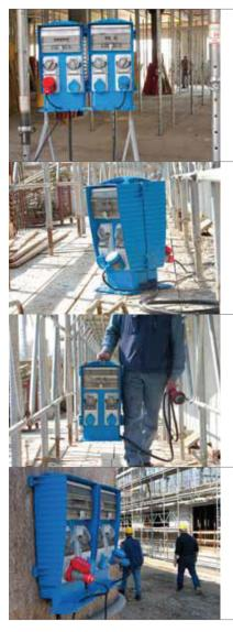
The front lid allows the operators to access to the board protections any time in any place it is installed.
